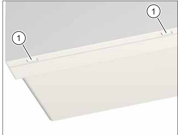
Fig. 25: Removing the cover from the ventilation unit
